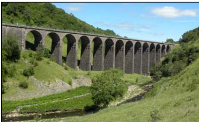
The old railway viaduct built with Ashfell Sandstone, across Scandal Beck within Smardale Gill.
